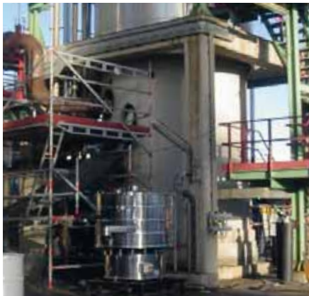
Sieve shaker for granulometric separation at a chemical plant, installed outdoors for raw material recovery. FTI-1500 sieve shaker with four simultaneous separations.
